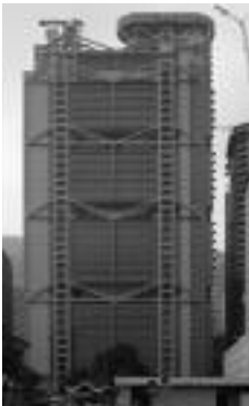
4.1. Banco de Hong Kong y Shanghai, Hong Kong. Foster Associates, 1986. Fachada principal.
